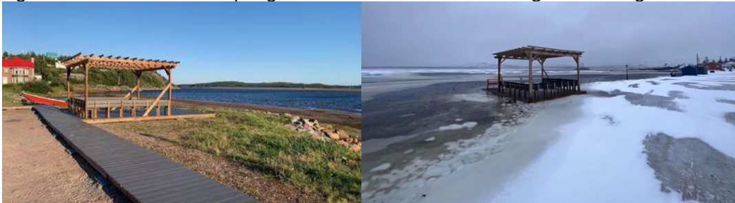
Figure 10: River before the spring 2022 flood that caused flooding in Saint-Augustin
